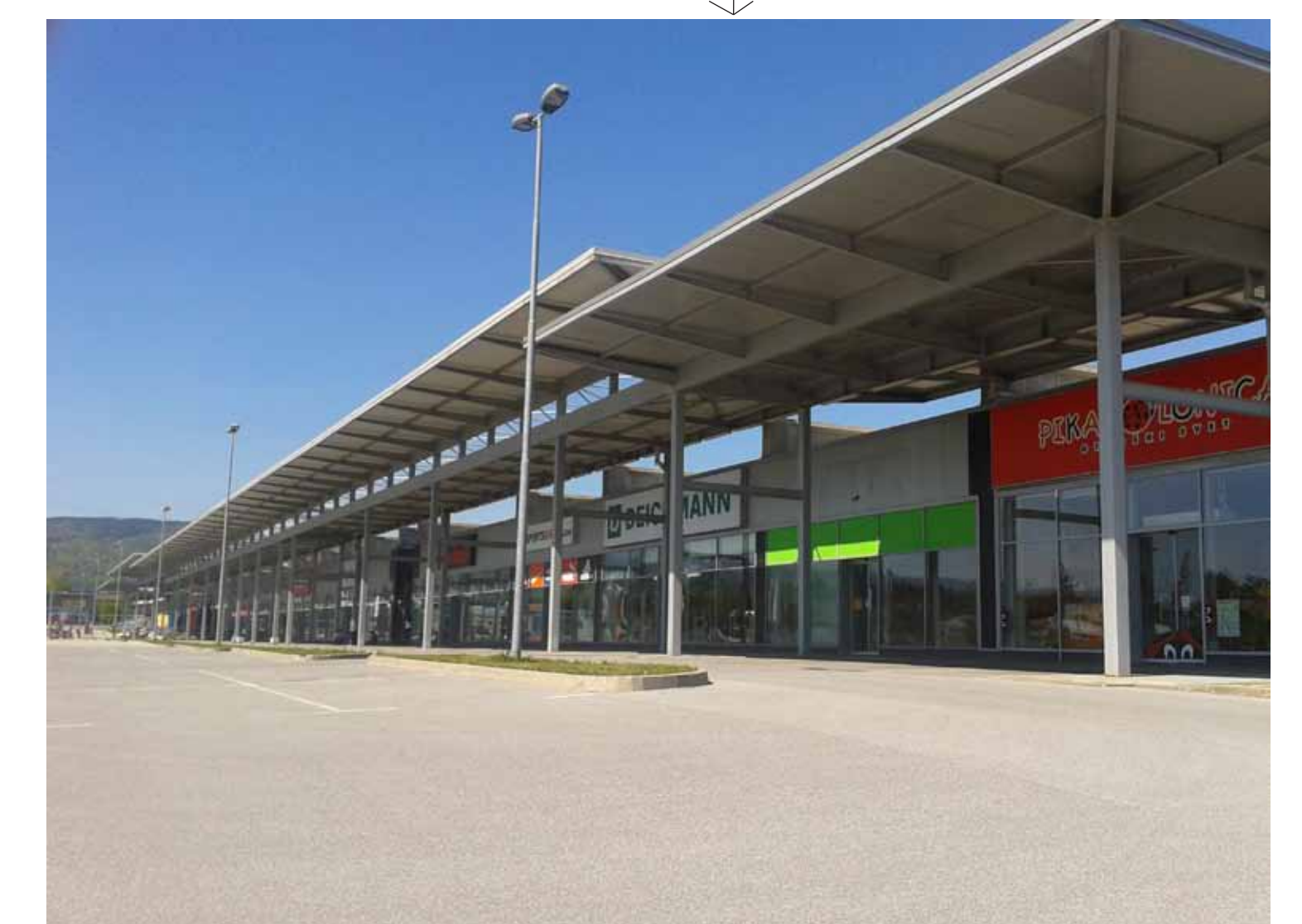
The shopping centre was built during the period from 2003 to 2011.
