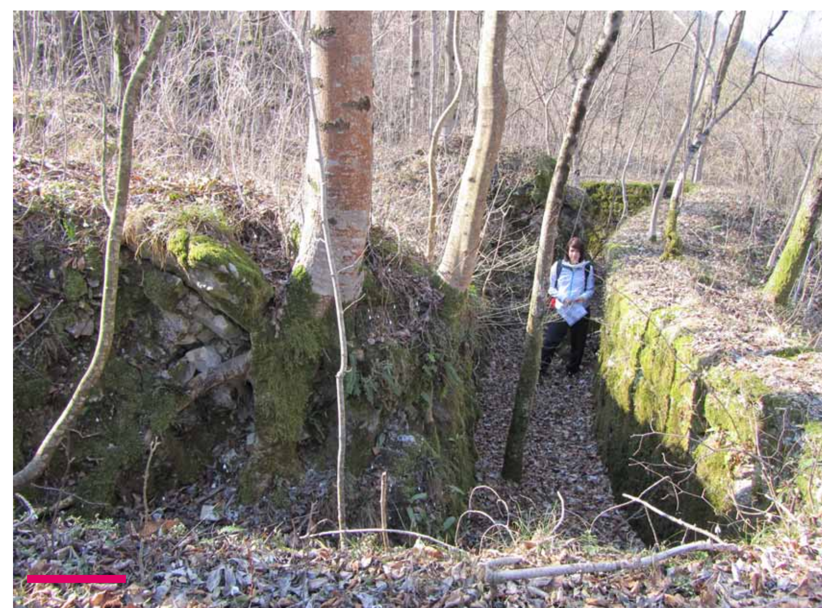
Accuracy of the engineers at building high trenches, which were covered with corrugated iron, can be seen.
