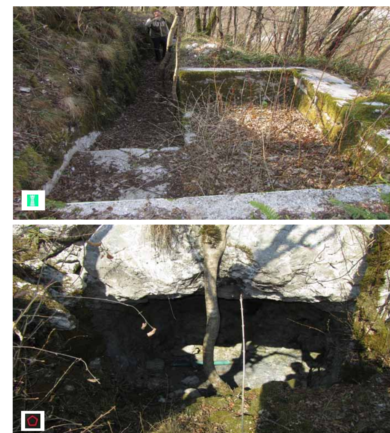
Above: A shooting position is connected with a trench. A concrete plateau was probably used for small arms. Below: A bunker on the south side of the hill with the view to Furlania. It was used as a observation point or as a shelter.
